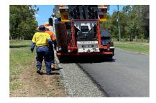
Edge break repairs are a breeze with cabin control of rotary broom stone / spray selection. Operates on both left and right hand side for increased application.
