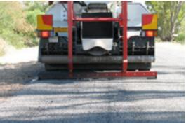
Road profile correction using full width adjustable screed bar.
