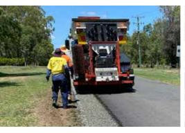
Edge break repairs are a breeze with cabin control of rotary broom stone / spray selection.
